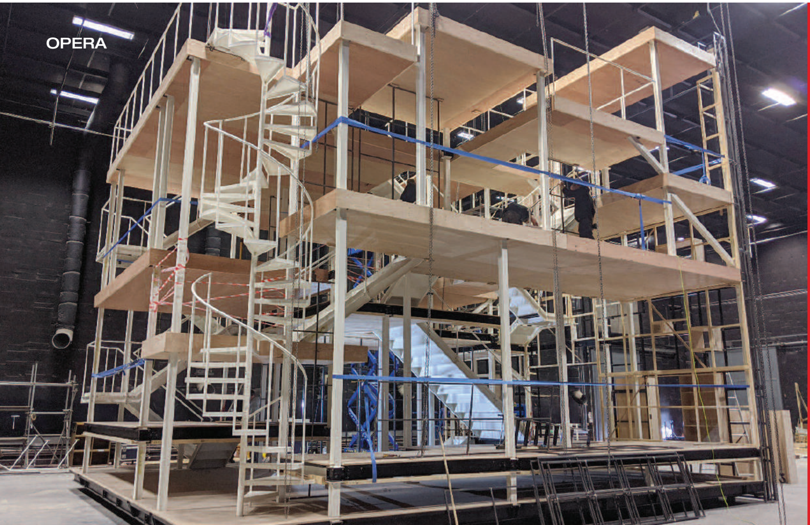
Martin's basic set, seen above, is a skeletal structure that is transformed by the addition of panels, as seen in the Vectorworks rendering, below right. The set was built by Bay Productions, of Cardiff, Wales.
